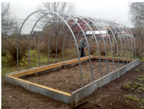
Picture12: Above Ground Foundation Wall
