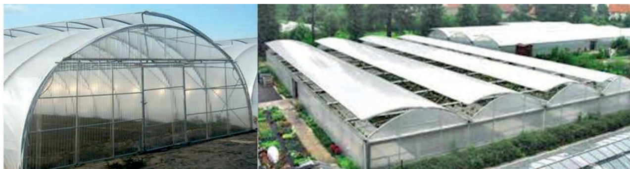
Picture 9-10: Individual and Block Greenhouses with Round Roofs
